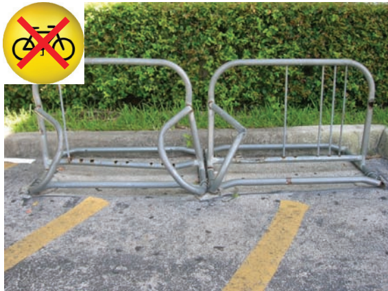
Fig. 39: A badly damaged, poorly maintained “comb” rack provides an inadequate, unsafe and unsightly bicycle parking facility.
