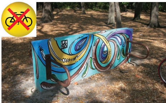
Fig.7: This public art bicycle rack is poorly located, inefficient, and does not provide enough frame stability for parked bicycles.
