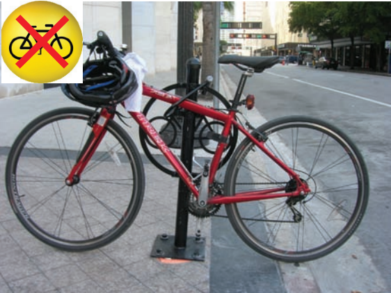
Fig. 21: The post and ring is a good rack choice, but as installed it places the bicycle in the motor vehicle right-of-way.
