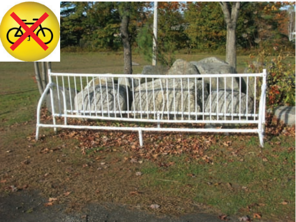
Fig. 28: This comb rack at the YMCA has already been damaged, and requires bicyclists to inconveniently lift their bicycles over the rack.
