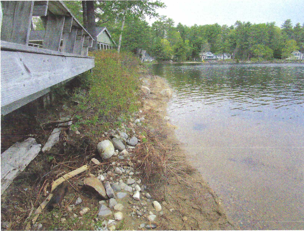
Photo 3. Close up view of the sweet fern shrubs on the shore that eroded from the bank during the heavy rain event on April 30, 2023.
