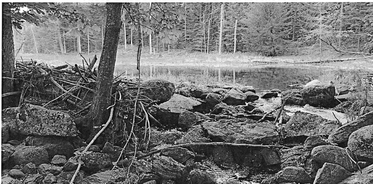
FIGURE 8 – PHOTO OF BREACHED UPSTREAM DAM PHOTO TAKEN BY ACADIA CIVIL WORKS IN JUNE 2021
