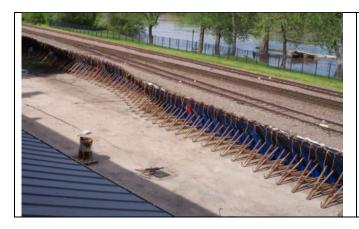
Porta Dam <u>Portadam | Decades of</u> <u>Water Control Expertise</u> Fabric covered braces used in construction as coffer dam
