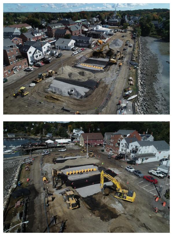
Although it appears that a large area has been graveled, there is still a need to maintain the construction barriers until the full stormwater retention system is installed. The construction foreman is eager to help restore parking as soon as he can for the business community. With that said, we may be able to open **a few parking spots on the east end of the lot for the weekend** as construction activities will break until Monday. A reminder that alternative parking
